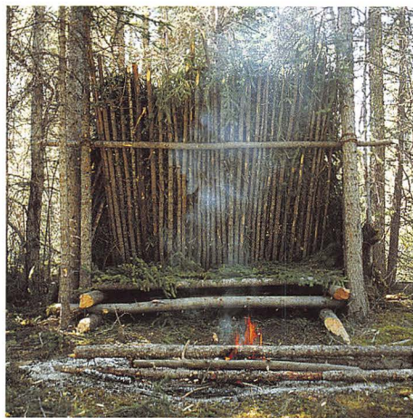
Classic northern lean-to in Rocky Mountains. Steep roof gives best rain proofing.
