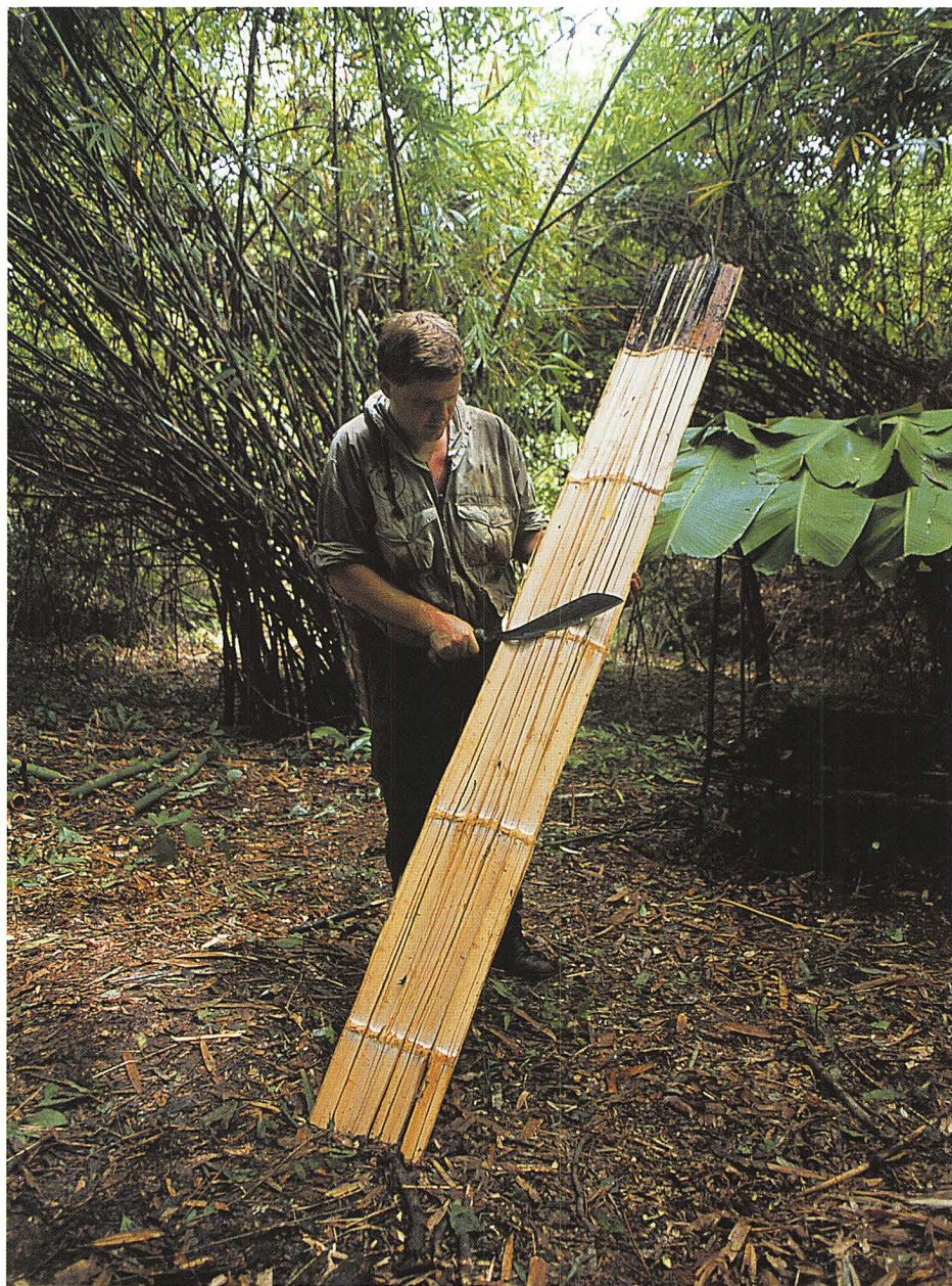
A parang must be strong and sharp to chop tropical hardwoods and to trim materials like bamboo, here having been flattened out for flooring.
