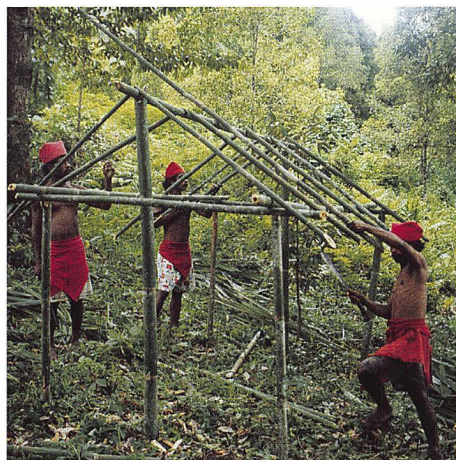
A strong roof design lashed together with sago palm midribs.
